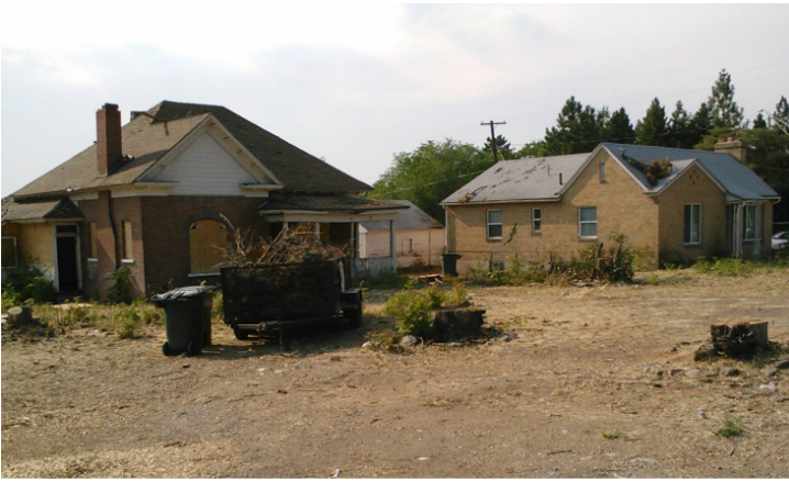
Existing Homes (to be demolished)
